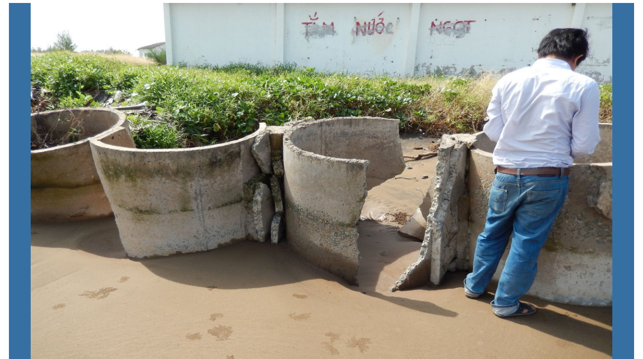
Figure 23: Damaged local erosion protection measures at site 3, eastern part
