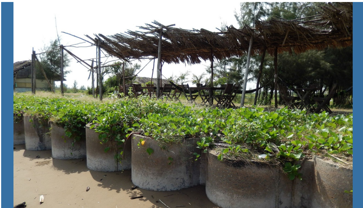
Figure 22: Local erosion protection measures at site 3, eastern part
