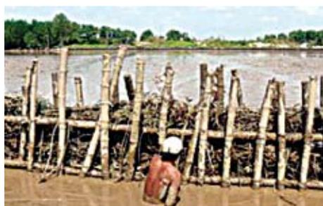
*Hold the line.* This is a static engineered response to shoreline protection using sea dykes. It should, wherever possible, be combined with mangrove protection and rehabilitation.
