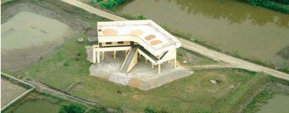
Photo; A cyclone shelter in the CZ
